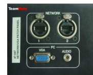
Example of column mounted patch panel for safe and secure connectivity
